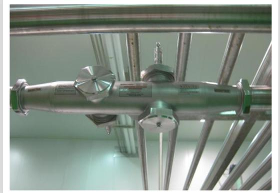
viscous pet foods and a large range of dairy products. The units can be Jacketed to allow for hot viscous products where required (e.g. chocolate transfer). The liquid pipeline magnet can be installed in either pressure or suction lines and is supplied with wetted parts of 316 (or special alloys for highly corrosive products).
